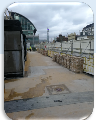
Image from roof above the hotel
